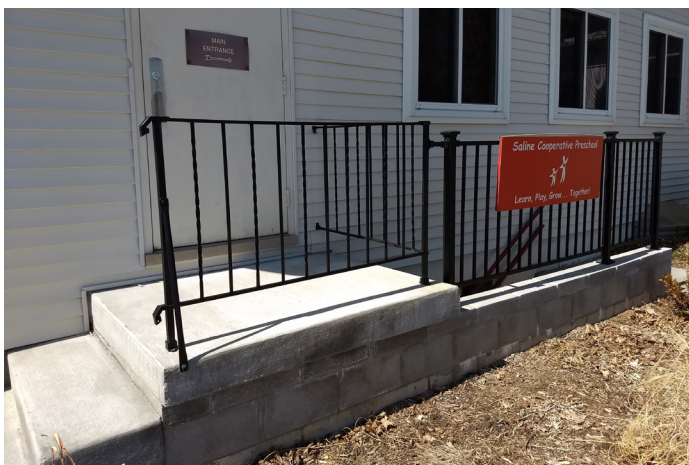
New concrete steps
